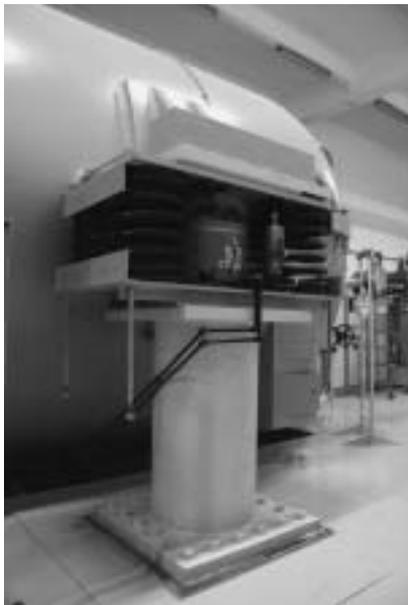
**Figure 2.** View of one of the four tank supports, part of the tandem earthquake protection system, equipped with an elastic GERB unit with springs and viscodampers.
